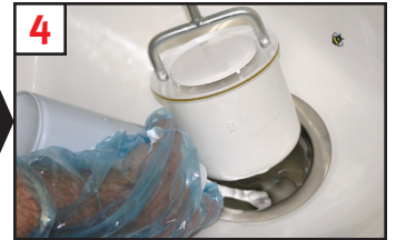
4 Lift and tilt cartridge to drain all free liquids then spray Falcon Foam Cleaner** into housing
