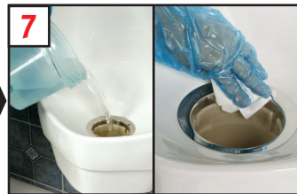
7 Flush housing with 5 gallons of hot soapy water then wipe clean inner stainless steel rim
